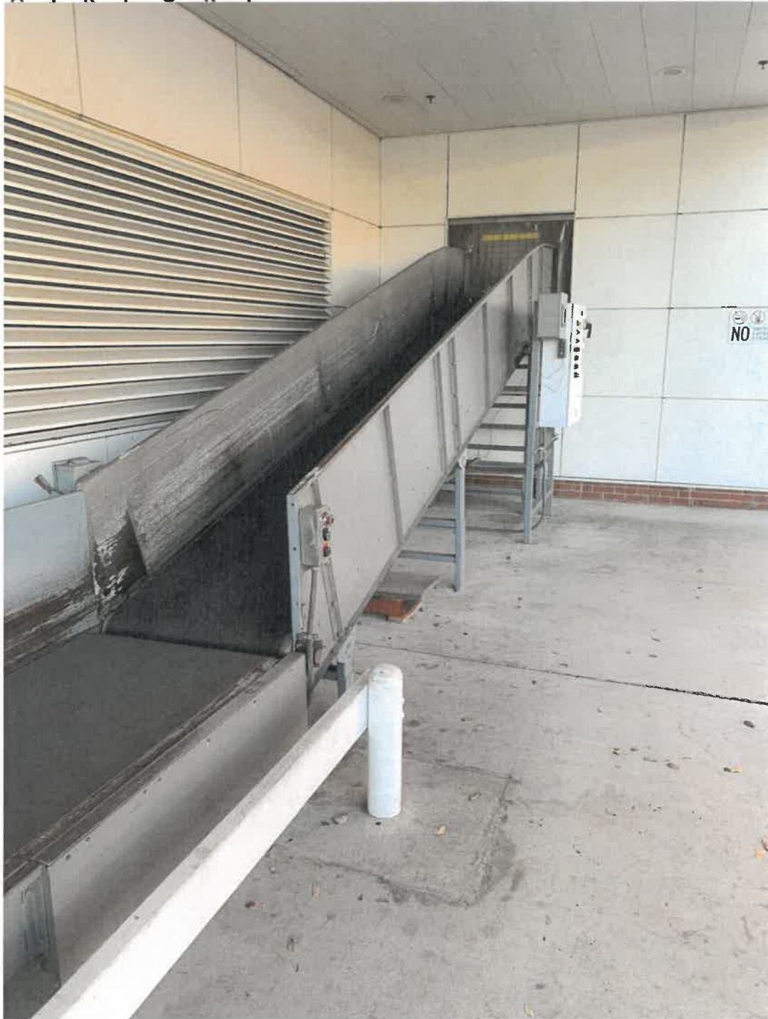
Incoming baggage drop off conveyor to carousel.
