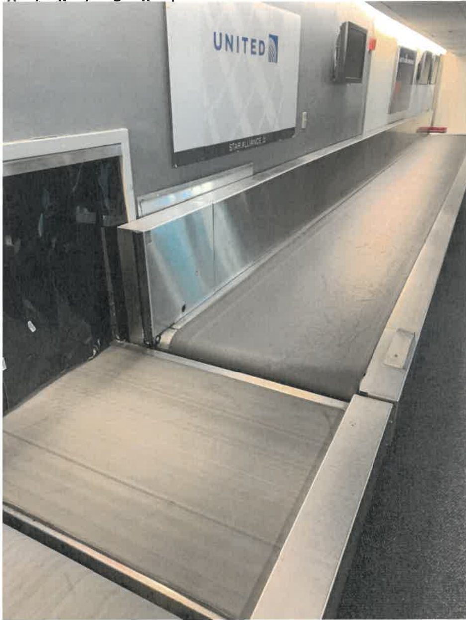
United/Delta Outbound baggage belt to tunnel.
