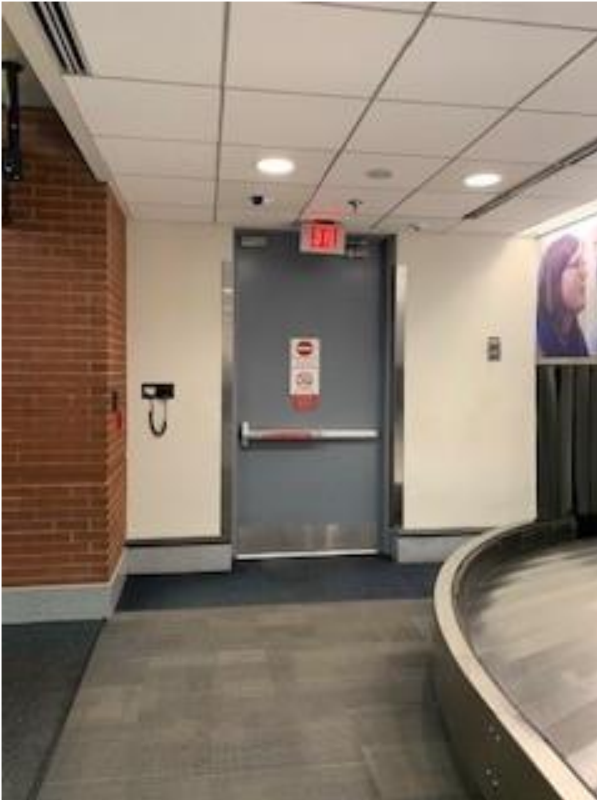
Departure Doors – Add-on Alternate Single manual door at southside of Baggage Claim Area
