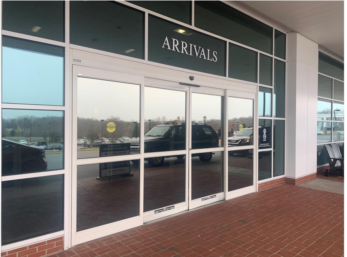
One of Three Sets of Automated Terminal Entrance Doors – The view is from the curbside looking toward the terminal.
